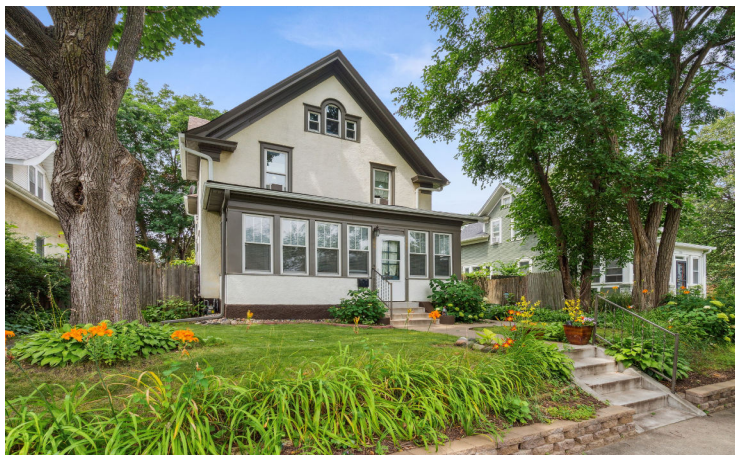
With new roof, gutters, windows and boiler, the big stuff has been done to keep your expenses down
