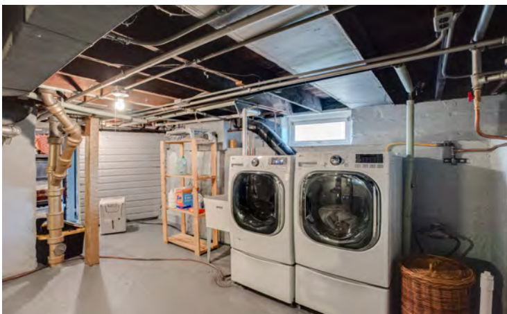
Full, clean basement with new front-loading washer/dryer and utility sink
