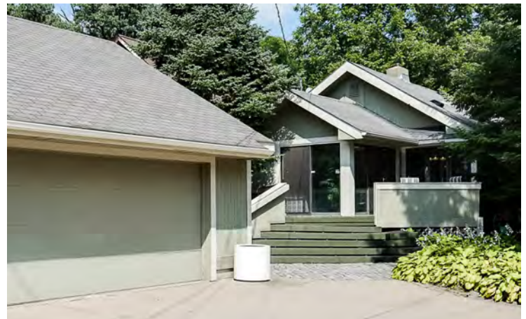
The well insulated garage keeps temperatures about 30 degrees higher or lower than outside.
